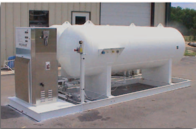
Propane tank on a movable skid.
